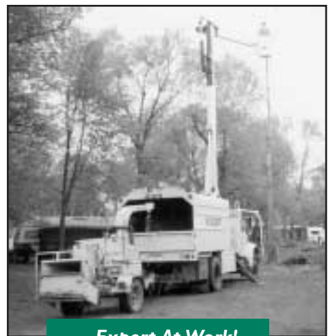
Minnkota Division Trimmer Dave Hanson starts to fell a towering Lombardy tree away from a 69 KV line.
