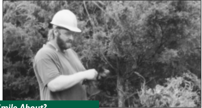
WTS cleared out the access to a power line. In right photo, Trimmer Jason Patterson slips on his gloves, preparing for action (see story in News from the Branches).
