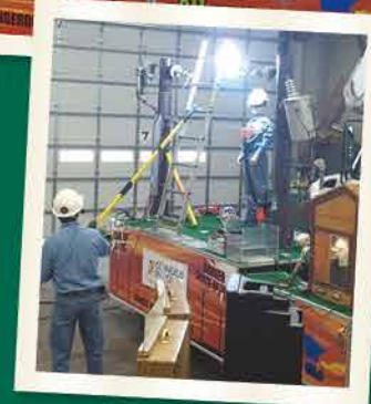
▲ Live line demonstration conducted by Connexus Energy
